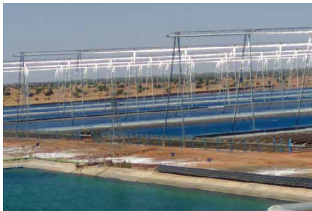
Figure 2: Reliance CLFR plant during operation at Dhursar
