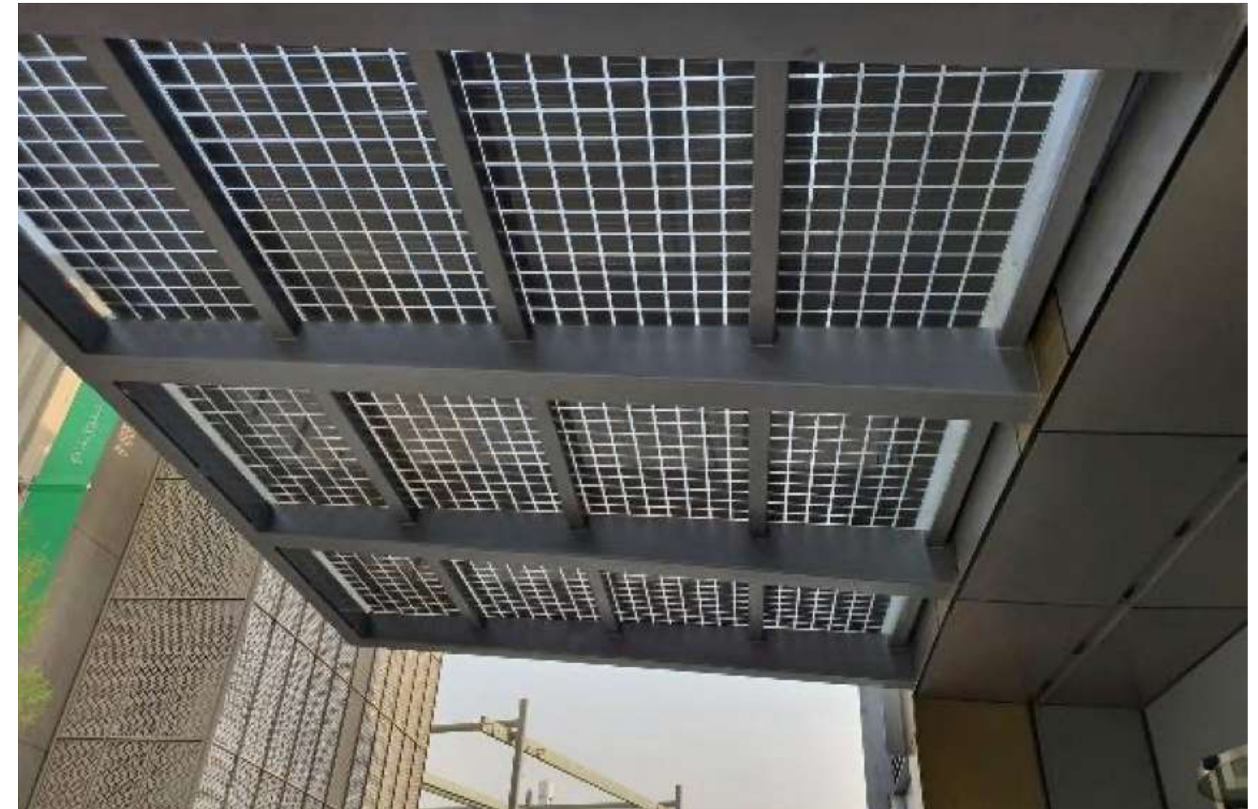
Custom solar canopy; hidden wiring and invisible mounting solutions
